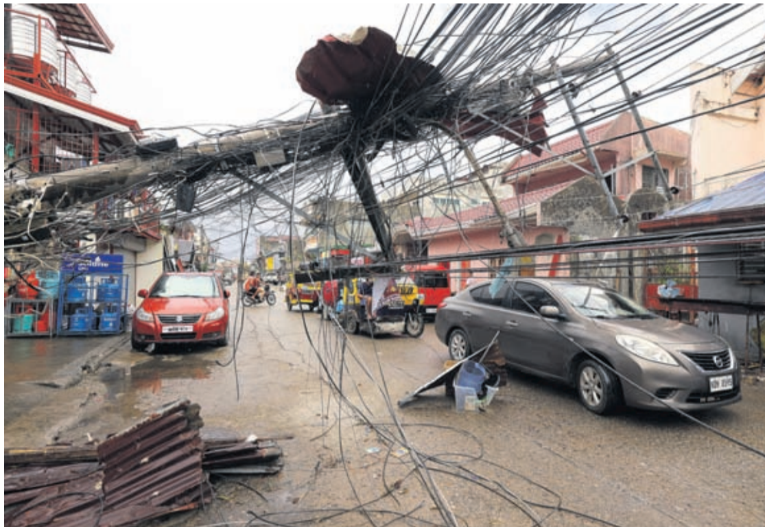
In this photo provided by Greenpeace, cars pass by a toppled electrical post due to Typhoon Rai in Surigao city, Surigao del Norte, southern Philippines as power supply remain down on Sunday Dec. 19, 2021.
